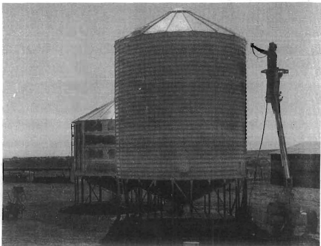
Fig. 4 Application of reflective coat to sealed silos.
